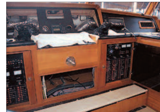
Careful preparation and effort results in holes measured twice, but cut once (above). The result—the completed pilothouse is both beautiful and functional (left).
